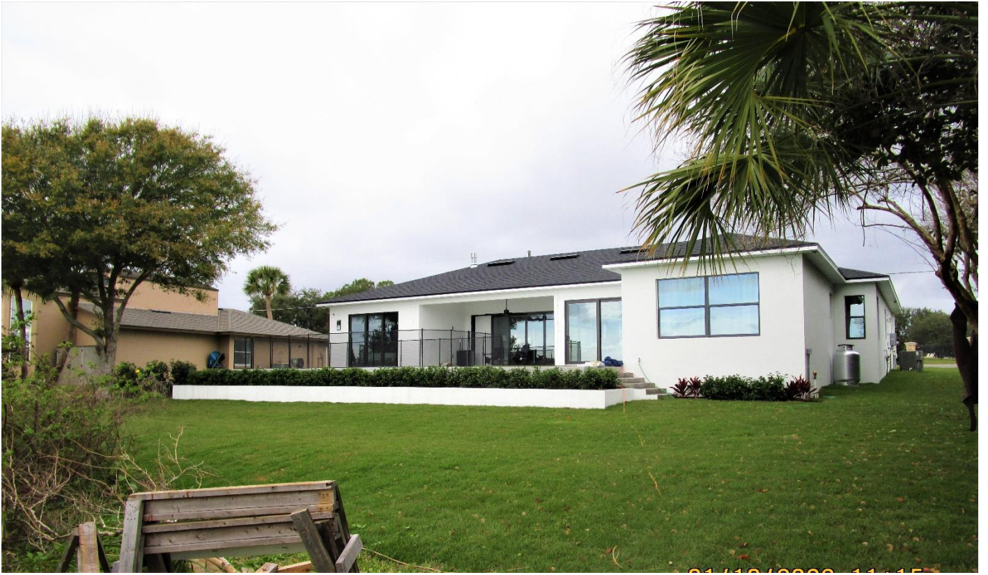
Rear yard, facing northwest towards pool and pool deck
