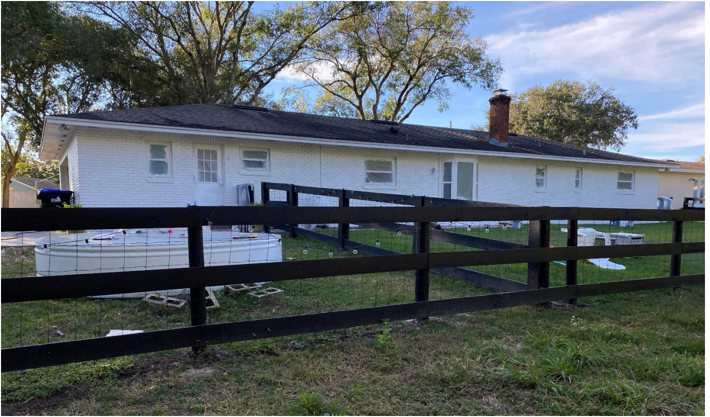
Facing west towards rear of subject property
