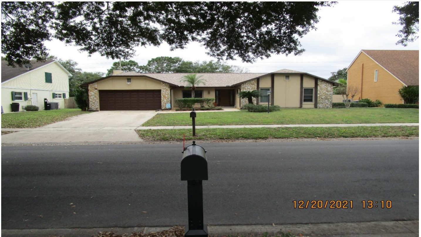
Front from Bonifay Ave., facing west
