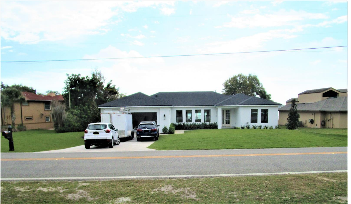
Facing south towards front of subject property
