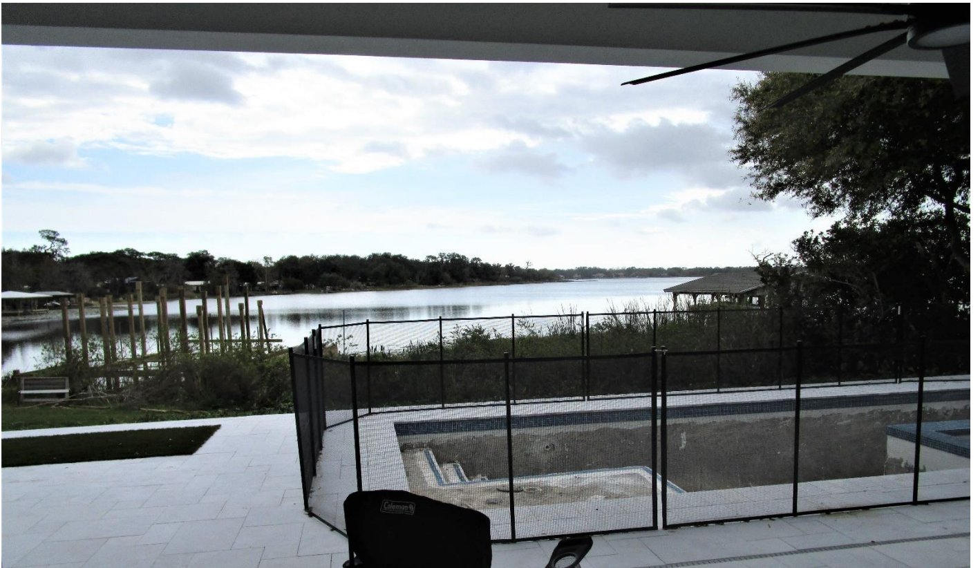
Rear yard, facing south towards Lake Crescent
