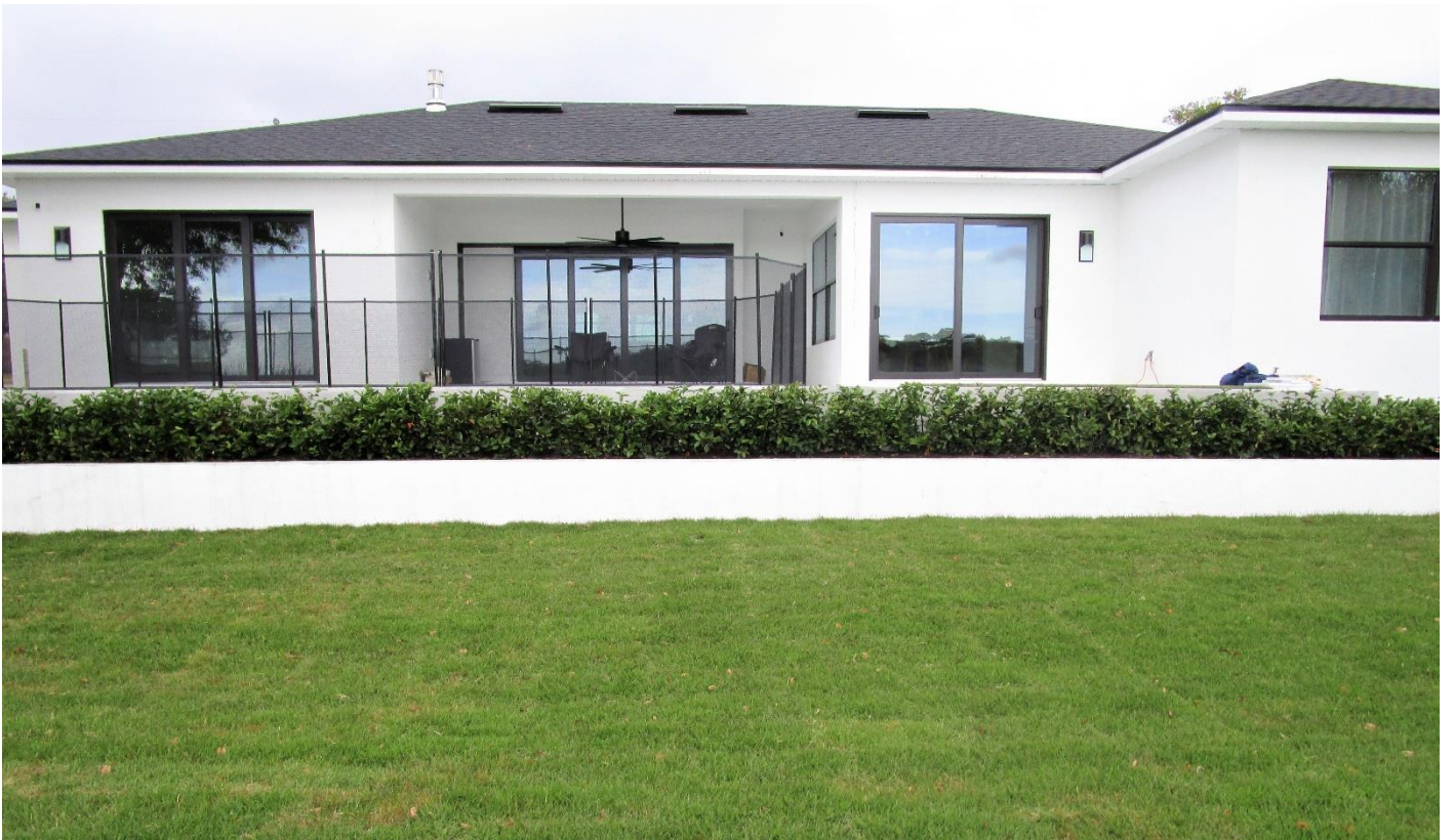
Rear yard, facing north towards rear of subject property (proposed screen enclosure)
