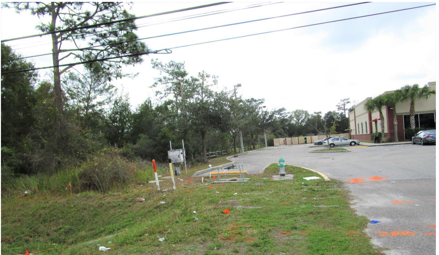
Facing south towards front side of subject property
